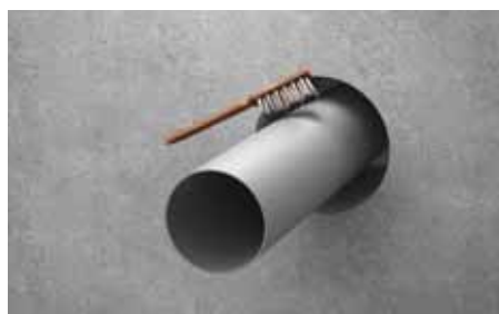
1. Clean the pipe and check the dimensions.
