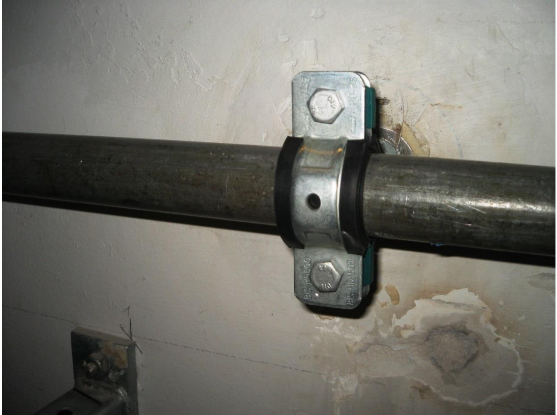
Fig. 1: Meas. 2: Heavy duty clamp BIS HD1501, 1" (30 - 35mm), connection M8/10, EPDM-rubber (30 x 4,00 mm)
