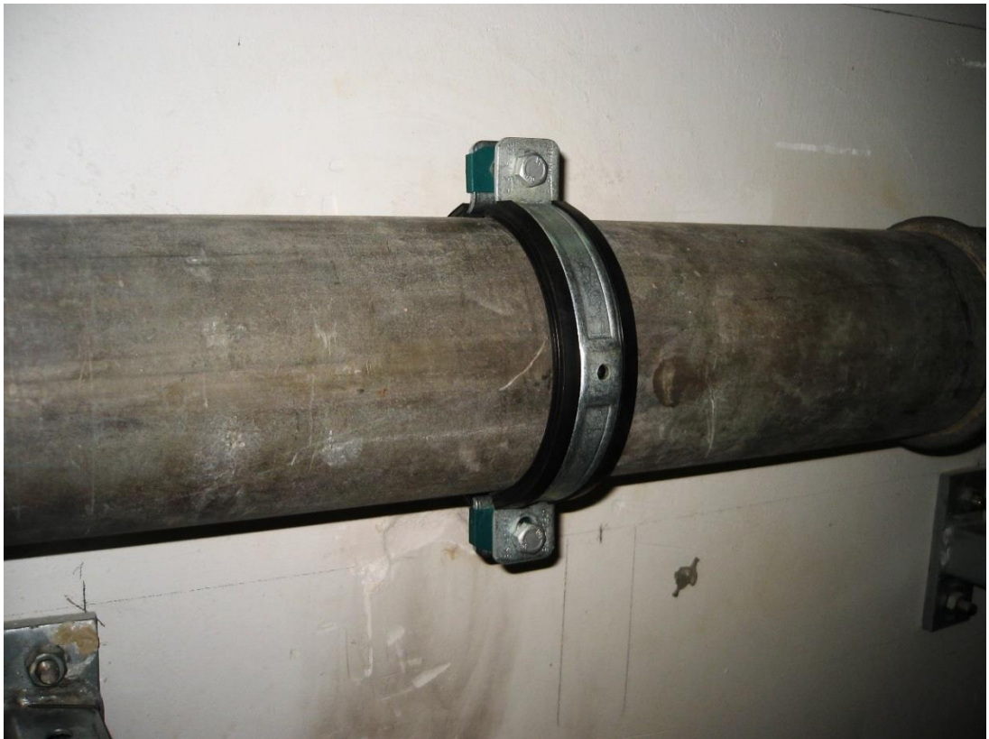
Fig. 2: Meas. 4: Heavy duty clamp BIS HD1501, 4" (108 - 116mm), connection M10/12, EPDM-rubber (30 x 4,00 mm)
