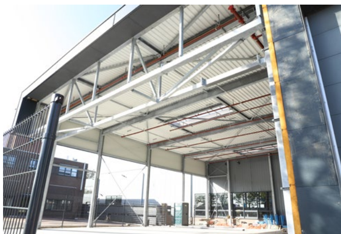
Truck loading dock - The Netherlands
